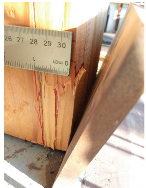
Chipping of wood at the rocking wall corner
