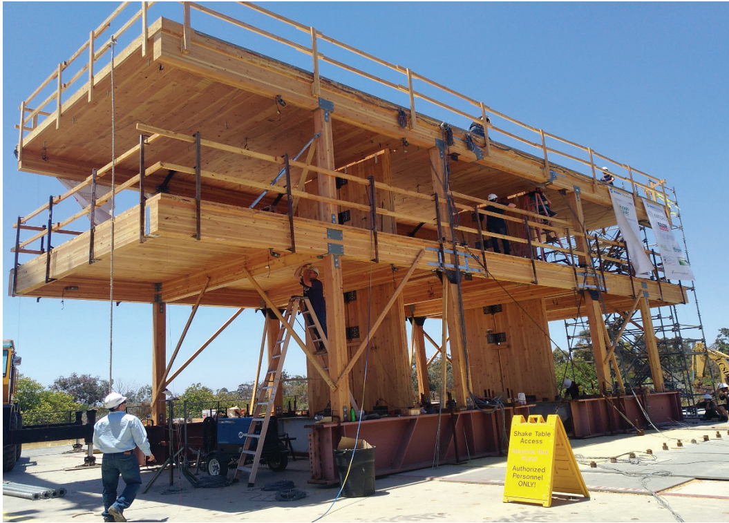
Figure 5: The test building completed with post-tension rocking walls
